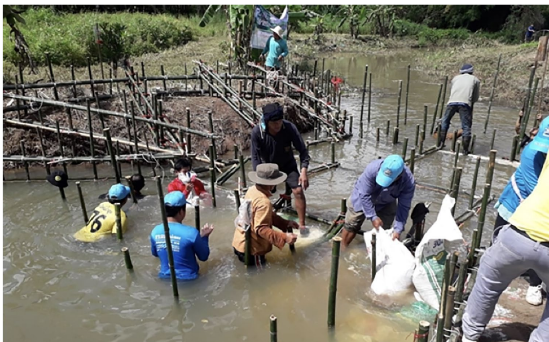
Figure 2 Living dam as a measure of ecosystem-based adaptation
