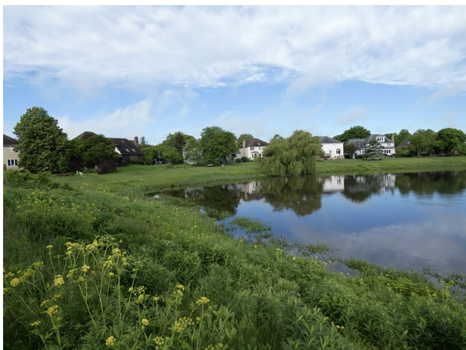
Figure 12 Temporary retention pond in a community
